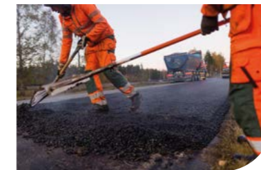
Construction materials and asphalt
